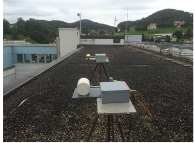
Fig. 3. Electric and magnetic field sensors on the roof of the Huber+Suhner building in Herisau.
